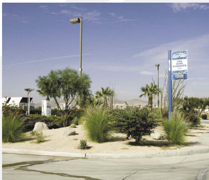
SunLine's fueling station site prominently stands out in Thousand Palms, California
